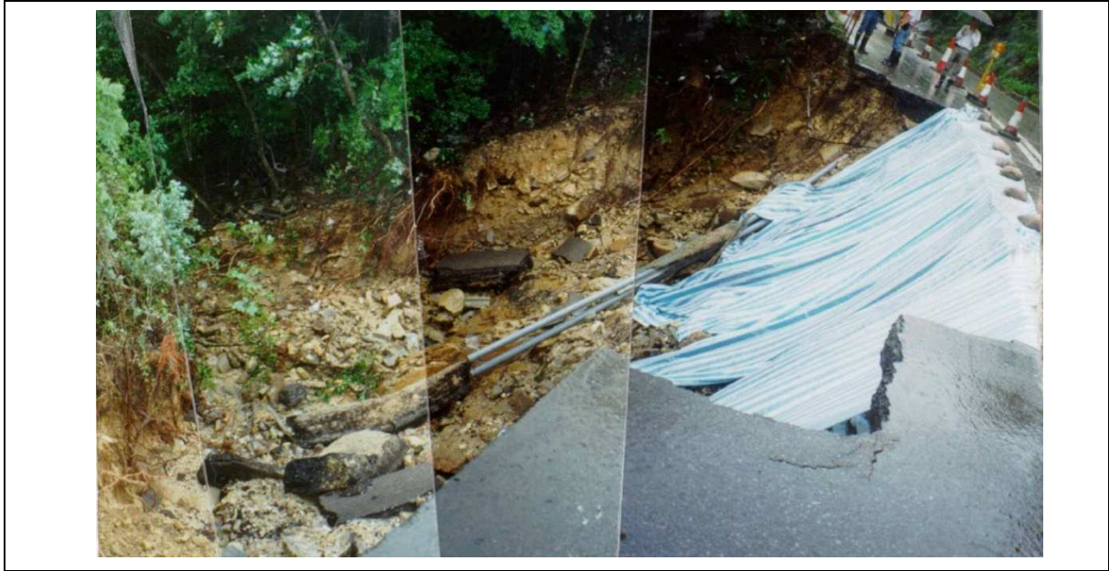
Figure 3.3 The 1995 Landslide (Photograph Taken on 13 August 1995)
