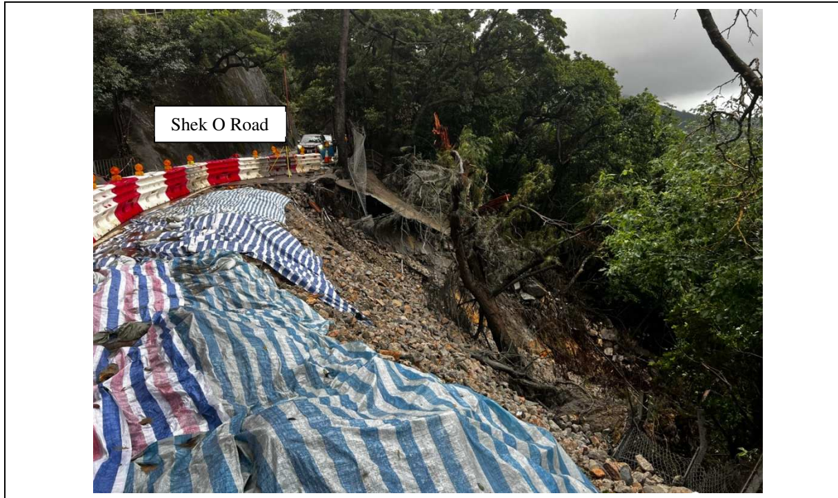
Figure 5.9 Rockfill on the Landslide Scar (Photograph Taken on 11 September 2023)
