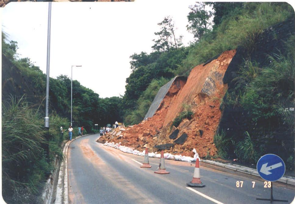
Description : Major failure of soil cut slope affecting road,
