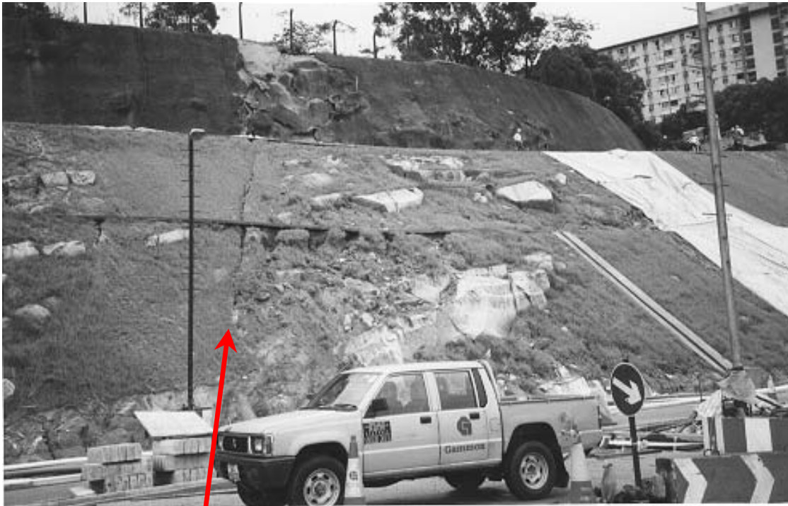
Discontinuity forming western release plane
