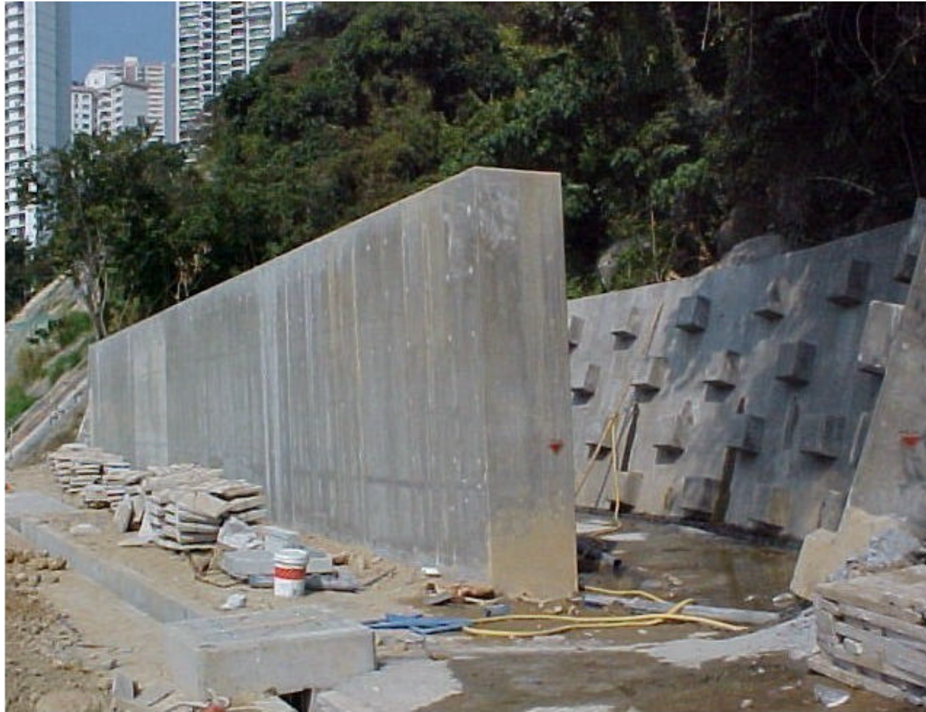
Plate 2 - Debris-resisting Barrier at Cyberport Development
