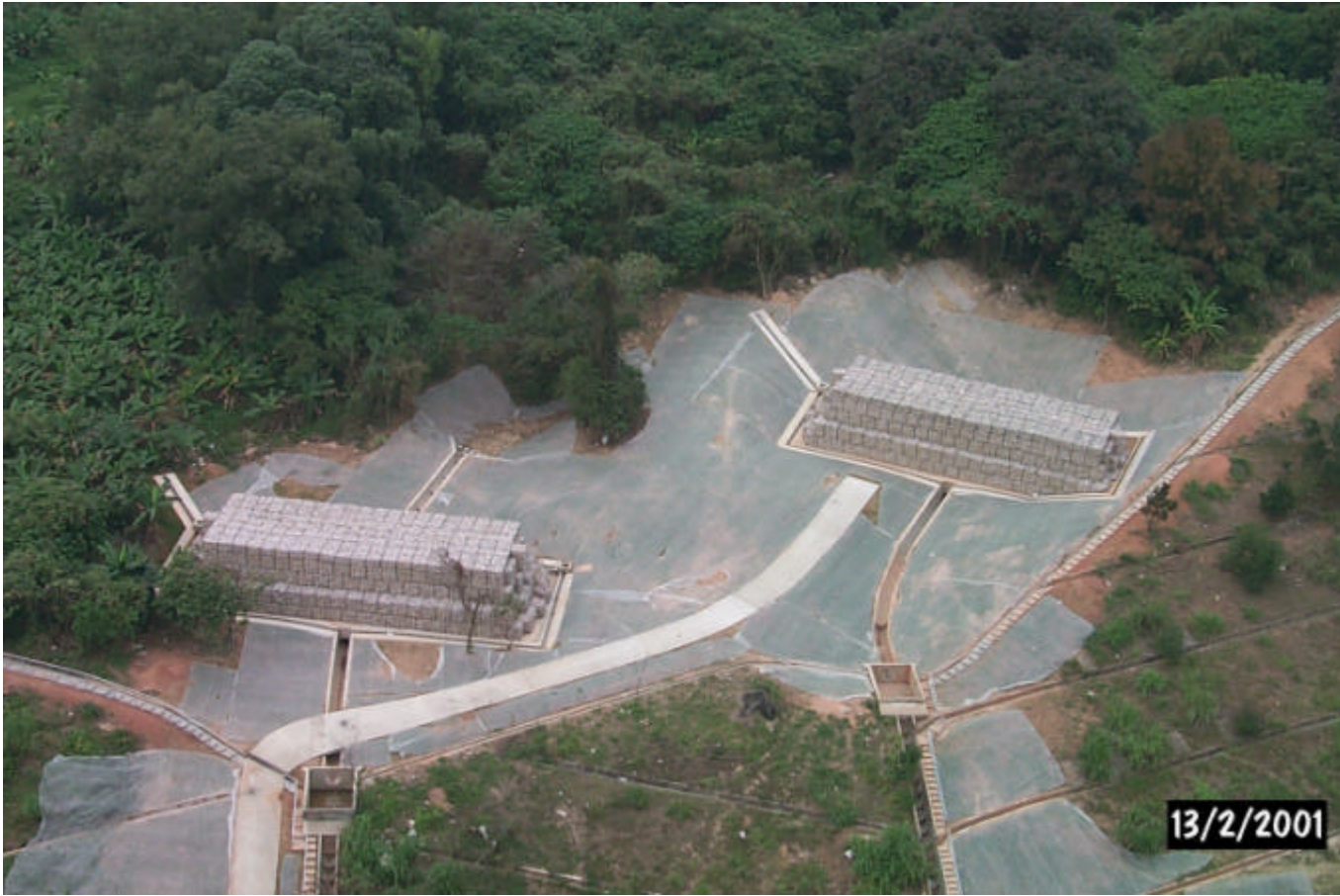
Plate 1 - Debris-resisting Barriers above Leung King Estate
