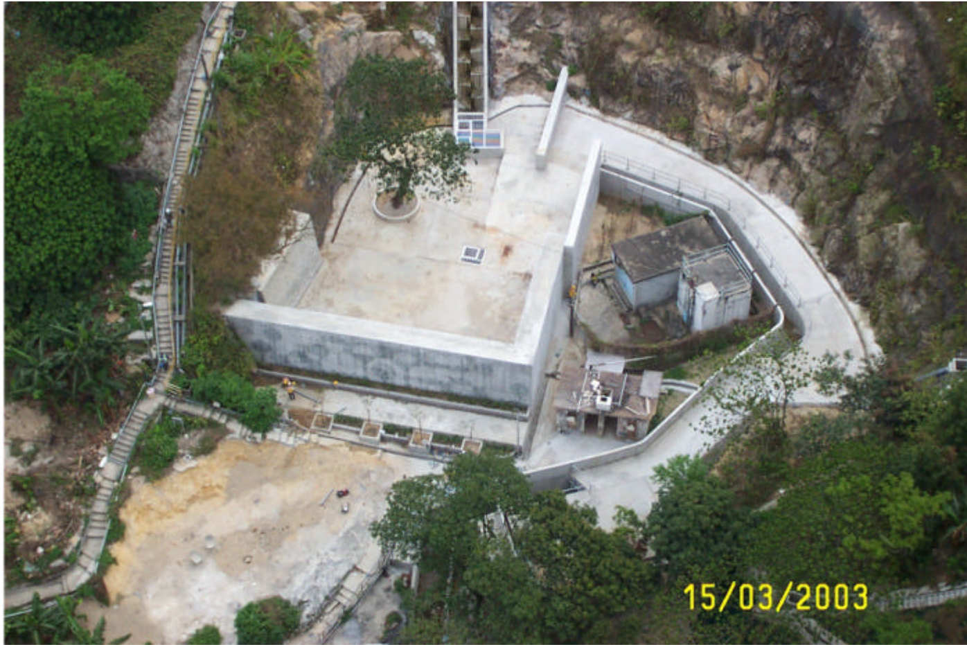
Plate 4 - Debris-resisting Barrier above Lei Pui Street
