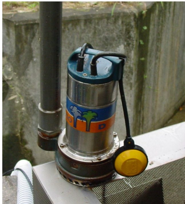
Plate 5 - Submersible Pump of the System
