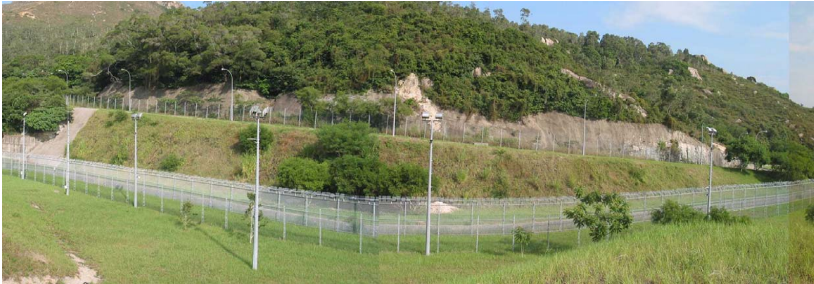
Plate 1 - General View of Slope No. 10SW-D/F75
