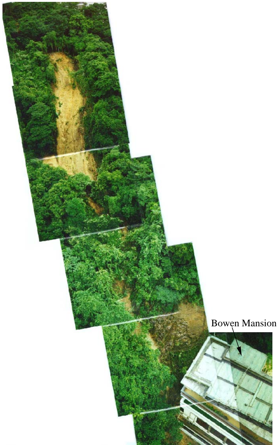
Plate 19 - General View of the Landslide - Bowen Road (Photograph taken on 11 June 1998)
