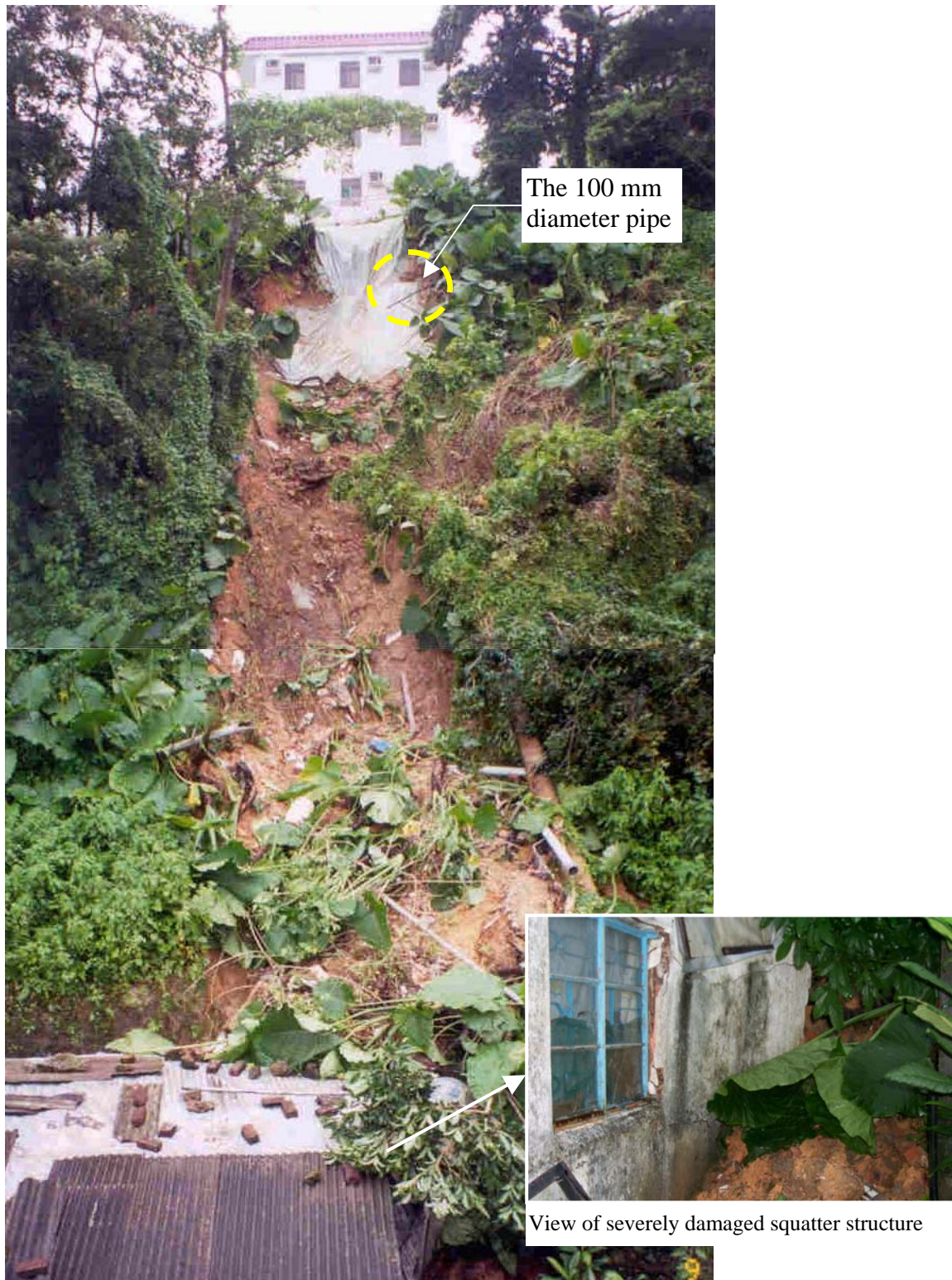
Plate 22 - General View of the Landslide - Denon Terrace (Photograph taken on 3 September 2001)
