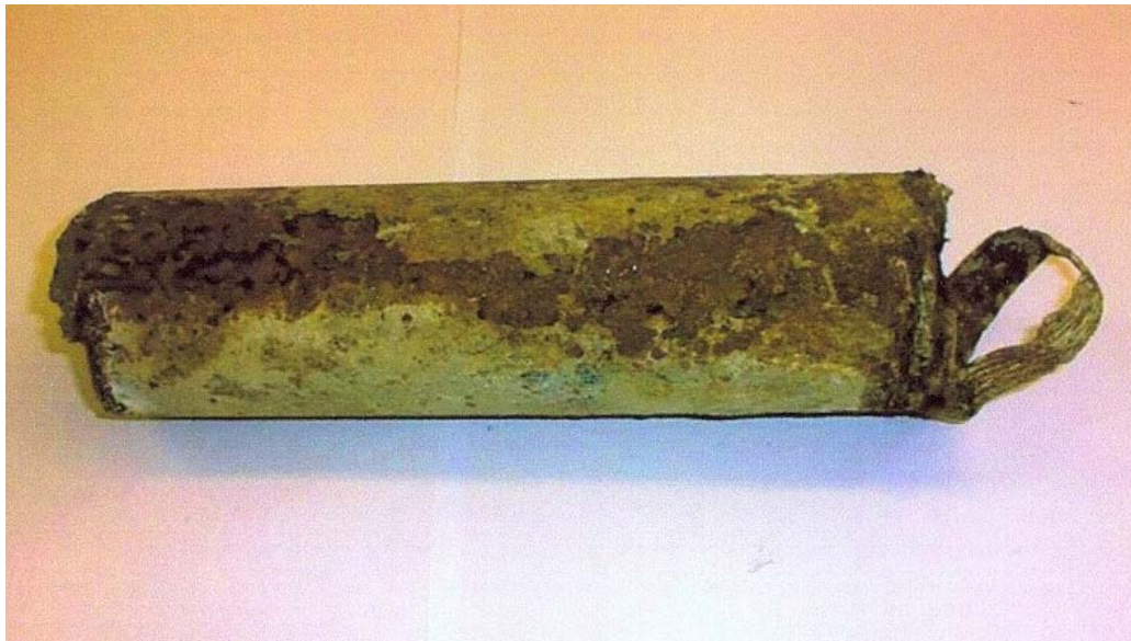
Plate 2 - Close-up View Showing Rusting Stains on the Underside of Pipe Surface - Hang Lok Lane (Photograph taken on 27 March 1998)
