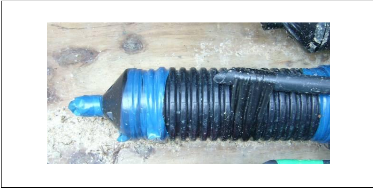
Figure 6.2 Sealed End Cap
